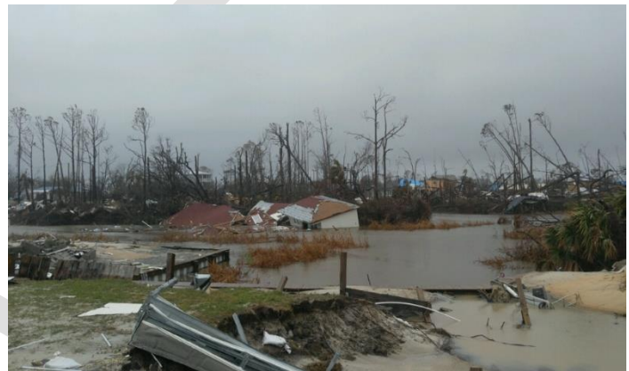
Figure 70. Extensive damage from Hurricane Michael in the back canal area. Source: City photo
