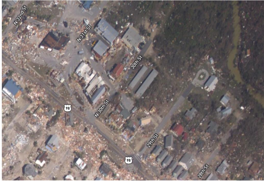
Figure 59. Damaged commercial area of the City following Hurricane Michael
