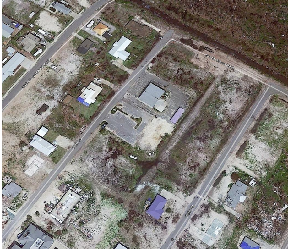
Figure 62. Aerial image of the Police and Fire Department facility and parking lot following Hurricane Michael
