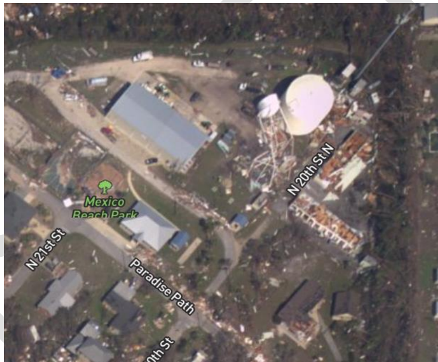
Figure 61. Topped City water tower following Hurricane Michael
