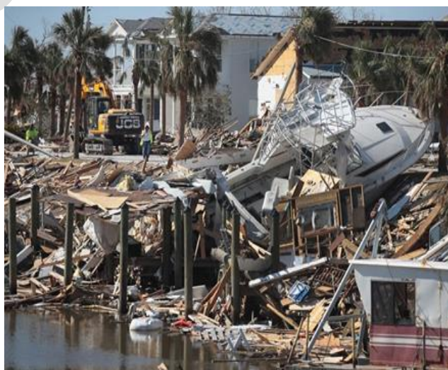
Figure 2. Extensive damage to the City Marina from Michael's storm surge. Source: City photo
