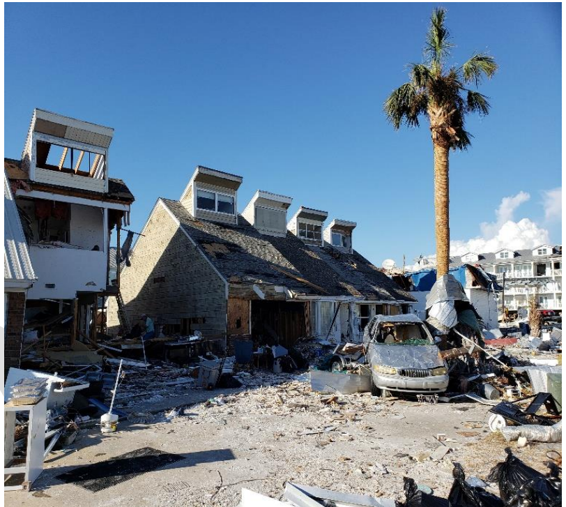
Figure 1. Post Michael damage. Source: Atkins staff photo.
