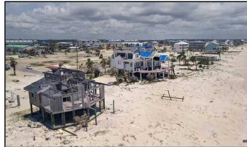
Figure 3: Property damage from hurricane Michael (2018)
