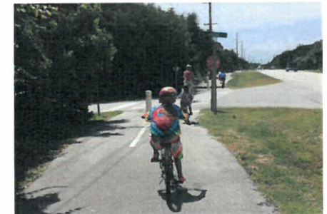
Shared dedicated path along two-lane highway with a grass swale.
