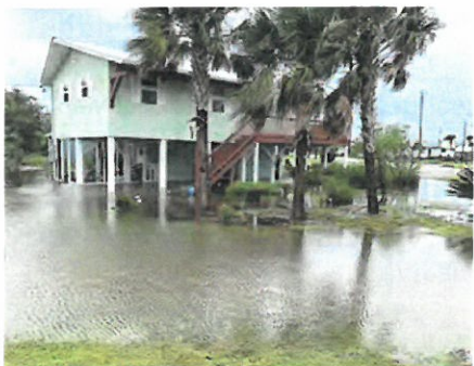
Recent flooding in the area.
