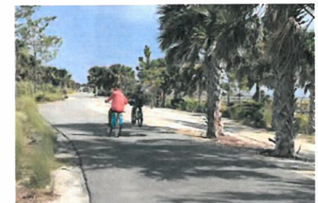
Local dedicated path with shoulders for pulling off or passing.
